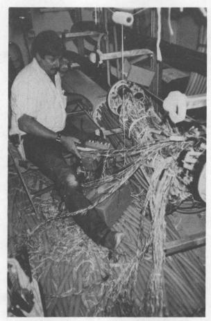
MICHAEL CROCKER, a US West employee, splices wires that will enable the Sandia telephone switch to connect its customers. The sight of 4,200 pairs of tiny wires might be overwhelming for most, but Crocker knows exactly where to connect every wire.
